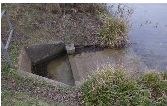
Photo 3 –Water overflow point for Balderton lake
